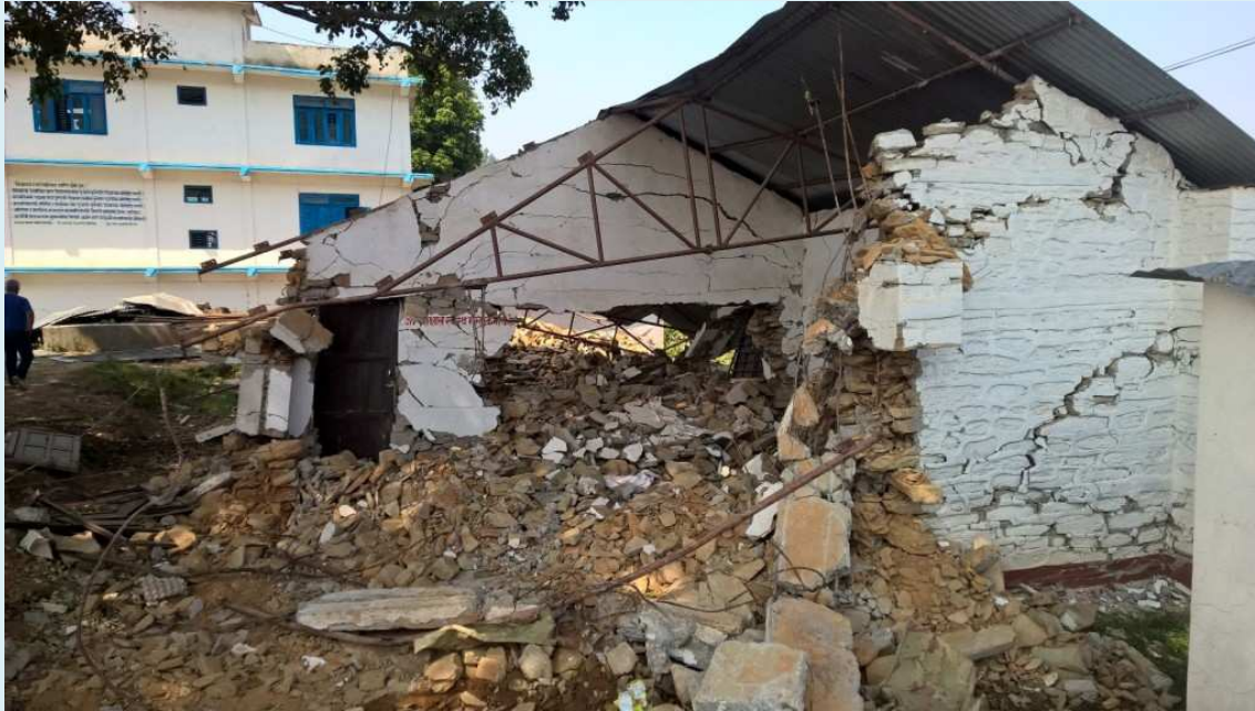
Destroyed Local Health Post & School Sangachowk, Sindhupalchowk
